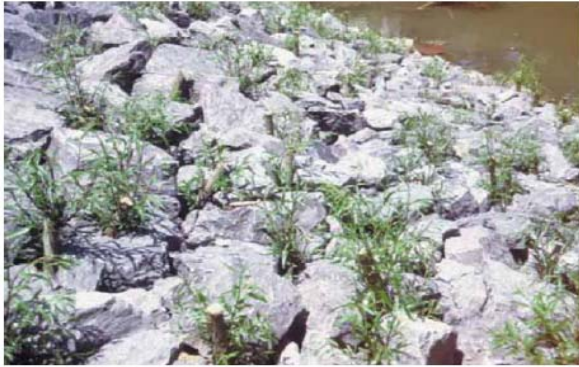
Vegetated Riprap along Stream Bank
