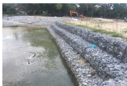
Constructed bank protection wall
