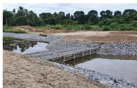
Constructed sediment detention weir
